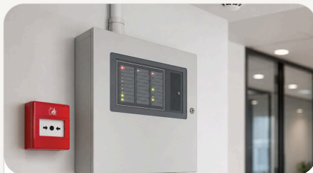
Conventional Fire Detection & Alarm Systems
